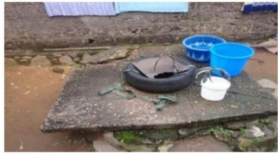
Figure 4: An Unprotected Hand-Dug Well in Ijebu Ode Town
